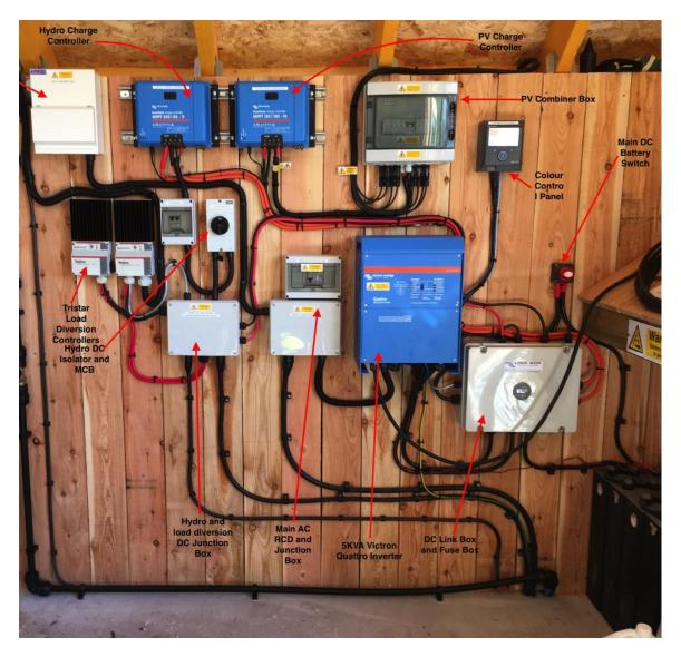
Victron has just introduced the 250VDC MPPT charge controller, which was installed here with a PowerSpout PLT85 without the need for any over-voltage protection. This is probably the first time the Vctron 250V controller has been used with hydro. Jamie can confirm that it works well.
